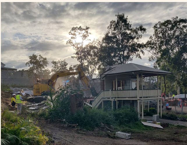
Image: Demolition at 29 Union Street, Taringa
